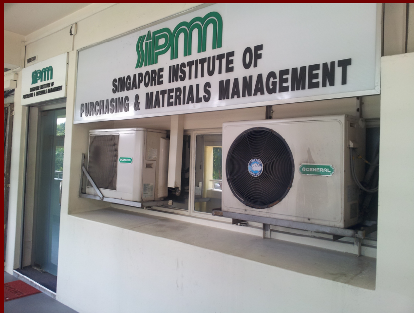
SIPMM Central Office (#03-3685)
